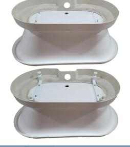
Check to make sure the spacers have not moved and are completely under the bracket. Fully secure the nuts to the bracket and tub with an impact drill and 17mm socket.
